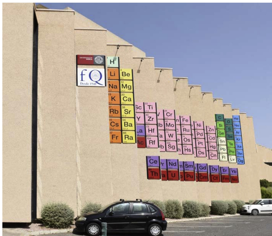
Fig. 1. Picture of the wall of the chemistry building in Murcia Spain.
